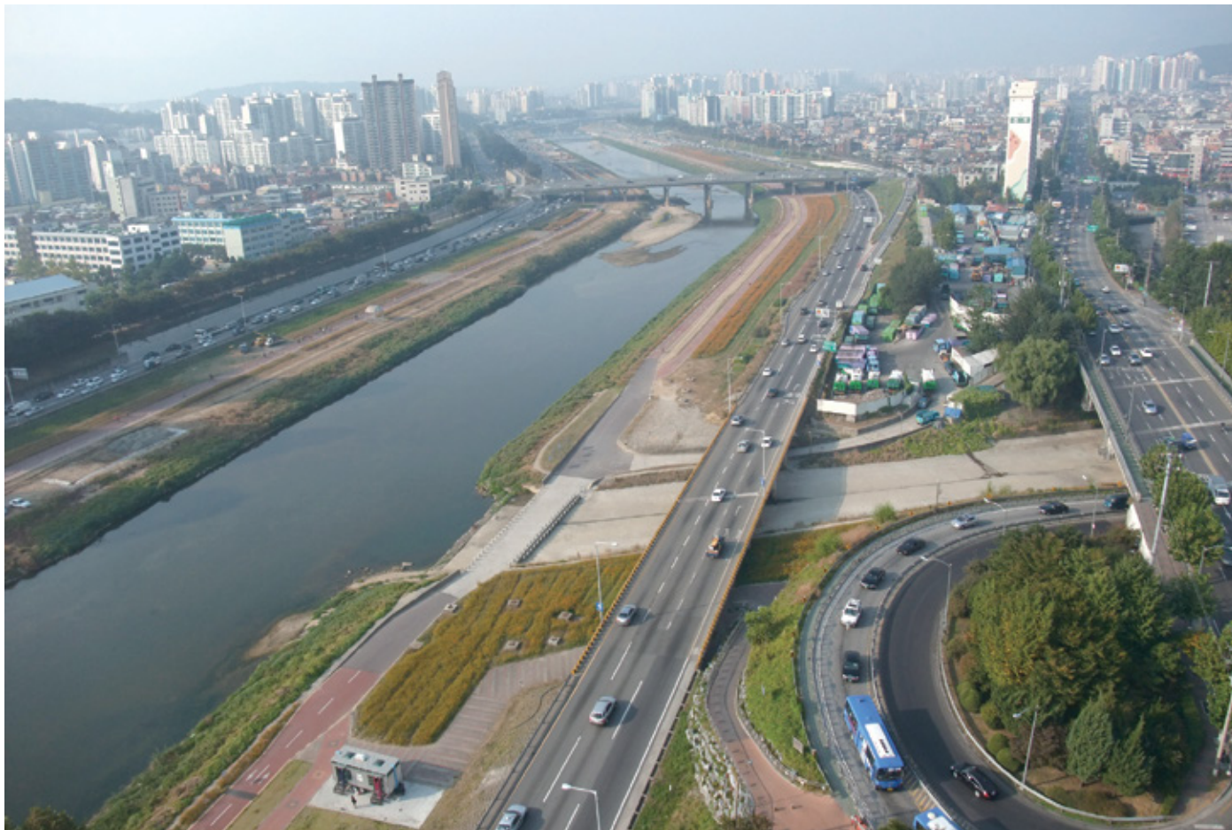
동부간선도로 침수 해소 공사 Constructed Settlement Work of Cumulative Flooding at Dongbu Highway
