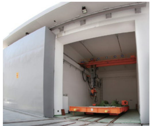
RT ROOM RT ROOM
